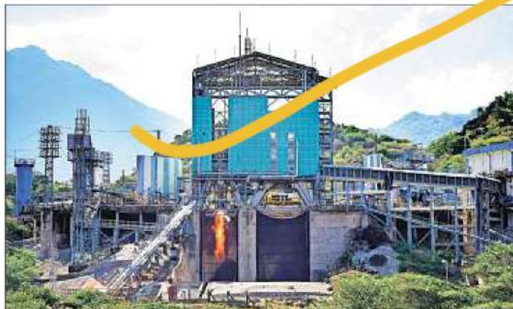
Flight acceptance hot test of CE20 cryogenic engine earmarked for the C32 upper stage of upcoming LVM3 mission at uprated thrust conditions of 220kN successfully carried out, at ISRO Propulsion Complex, Mahendragiri. (PTI)
