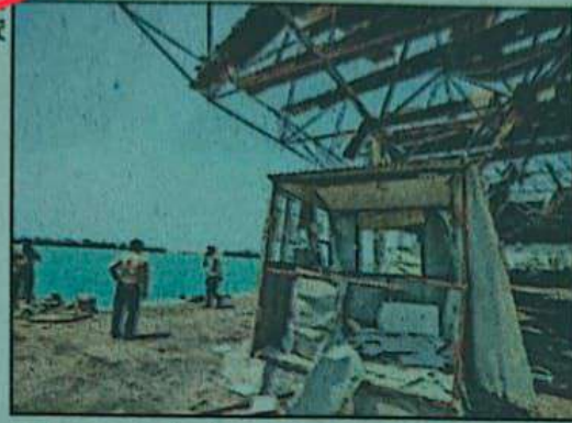
A damaged storage & warehousing facility at the port of Kuhestak in Iran's Sirik County Sunday, which was struck by the US military last week
