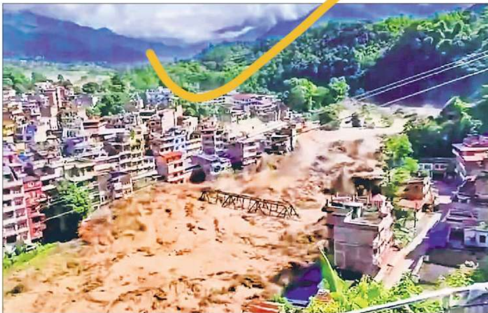
A video-grab shows a bridge being washed away as floodwater gushes through a residential area, in Nepal on Wednesday. (PTI)
