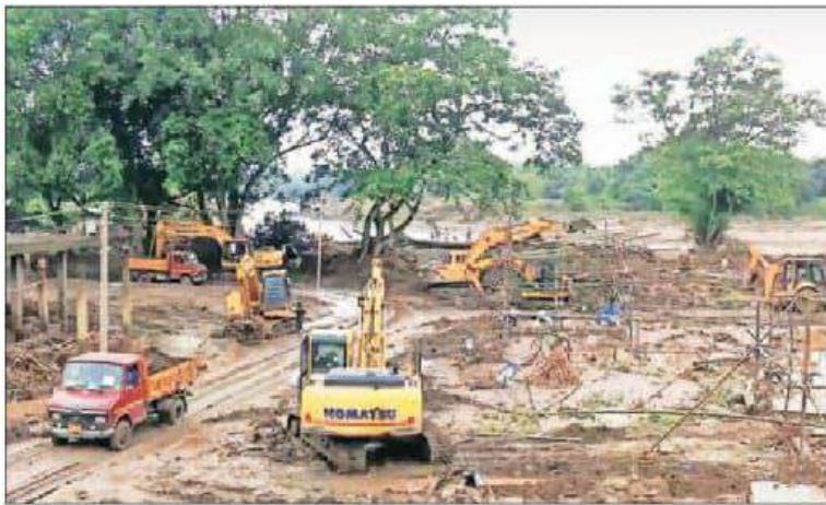
JCB excavators clear debris and scattered wooden logs which were swept away in a flash flood at Nepali Khuti area, in Sivasagar on Monday. (ANI)
