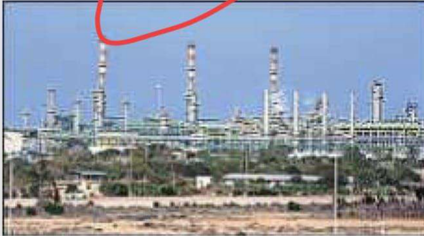
Mellitah Oil and Gas terminal.
