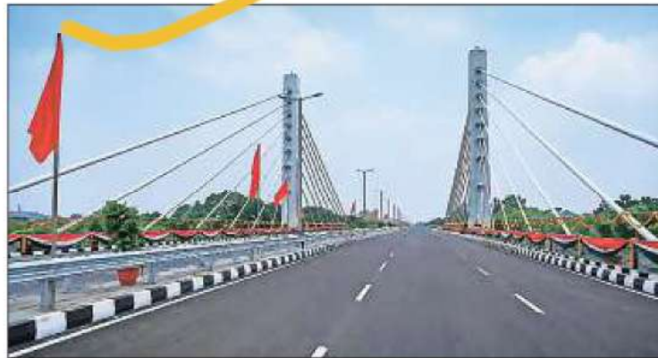
A six-lane cable-stayed bridge over the Narmada Main Canal between Koba Circle and Bhat Circle on the day of its inauguration, in Gandhinagar, Gujarat. (@CMOGuj/X via PTI)
