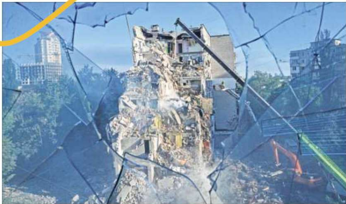
A residential apartment building is seen damaged after a Russian strike on Kyiv on Thursday. (AP/PTI)
