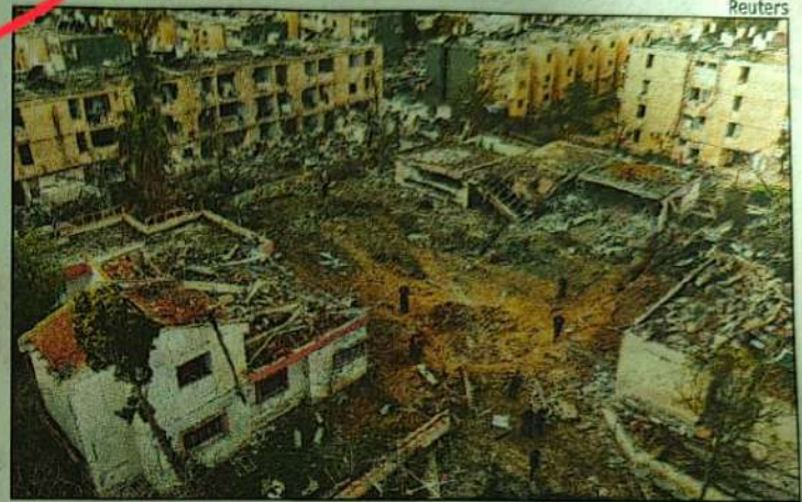
A drone view shows a damage in a residential neighbourhood in Dimona, Israel. Southern Israeli towns woke to widespread damage on Sunday after air defences failed to intercept two Iranian missiles overnight that injured scores of civilians in one of the worst attacks of the war so far on Israel
