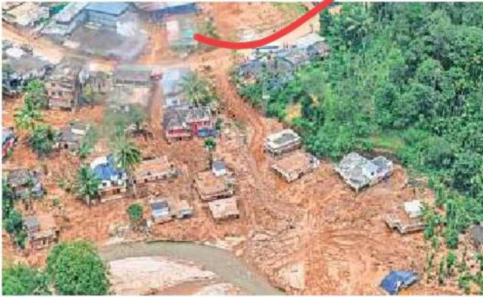
A view of the landslide-hit areas in Wayanad district on Saturday. (PTI)
