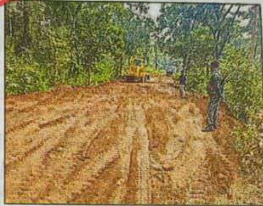
BRO has already started work in Maoist commander Hidma's den
