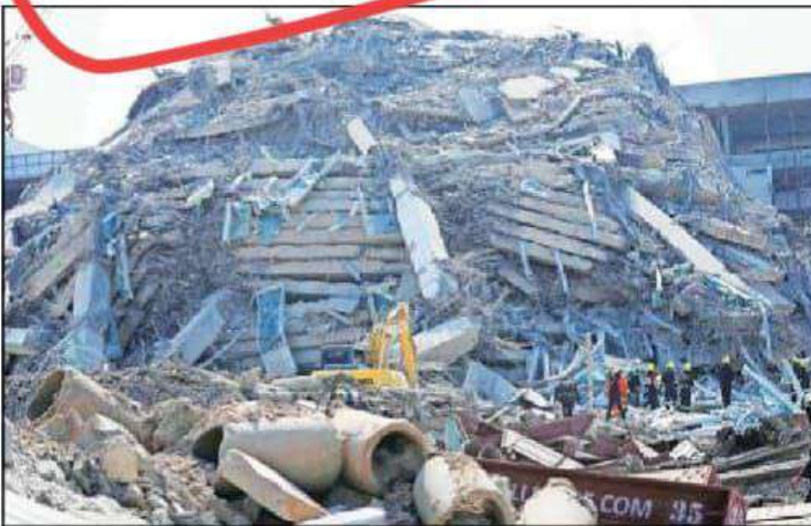
Rescuers work at the site of a high-rise building under construction that collapsed after a 7.7 magnitude earthquake in Bangkok, Thailand on Friday. (AP/PTI)
