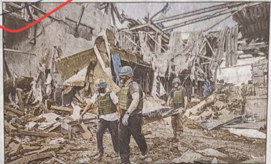
A destroyed Russian border post at Sudzha Border Crossing in Kursk
