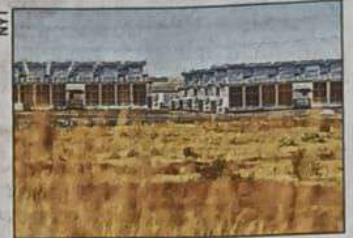
Citing surveillance & espionage risk, the bitcoin mine in Cheyenne, Wyoming, has been ordered to cease operations immediately
