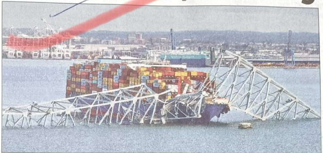
Dali crashed into Baltimore's Francis Scott Key Bridge, causing it to collapse and taking down vehicles and people. Six of the 8 workers who stopped traffic to the bridge after hearing the mayday call were missing
