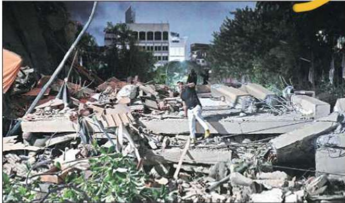
A man jumps on a collapsed building after an earthquake in Caracas on Wednesday. (AP/PTI)
