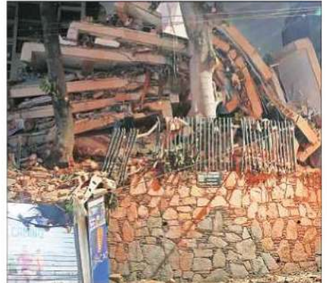
A collapsed building after an earthquake in Caracas. (AP/PTI)
